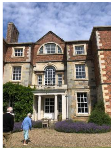
Boynton Hall, entrance.
