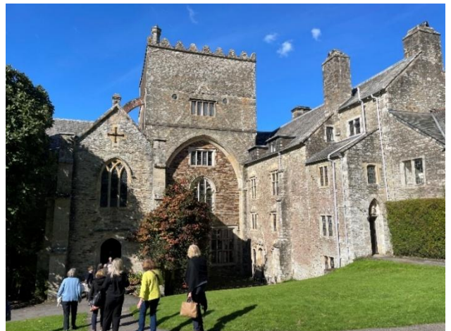
3 Buckland Abbey: exterior, showing the blocked transept arch and roofline of the former abbey church.
